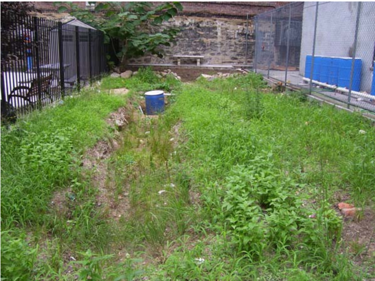
The barrel in the middle is a sump that controls the flow of rainwater form the rain barrels outside of the fence. Site still in development.
