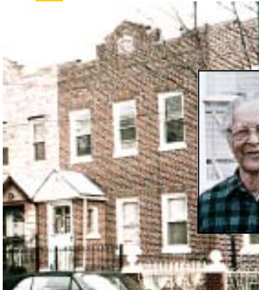
The Parodneck Foundation worked with Ms. Ruth Wells to create an assistance package that would rescue her home from predatory lenders. In the fall of 2002 Ruth Wells of obtained affordable re-financing and a SCHAP loan that covered the cost of home renovations including a new bathroom, kitchen, painting, sheetrock and electrical outlets.
